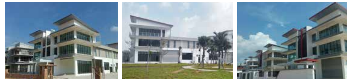
Senibong 88 construction in progress as of March 2015
